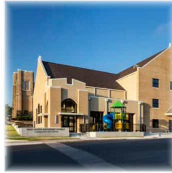
FIRST UNITED METHODIST CHURCH - HUNTSVILLE, TX
