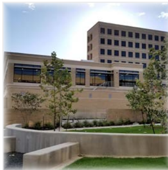
TAMU CONCRETE LAB
